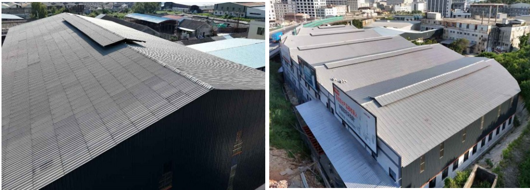
Figure 7 Corrugated sheet roofing of livestock building.
