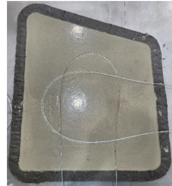
Step 3: Placing cable
