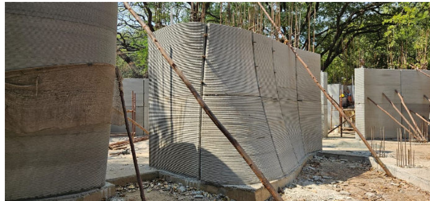
Guest house construction (3D concrete printing) IIT Madras, Chennai
