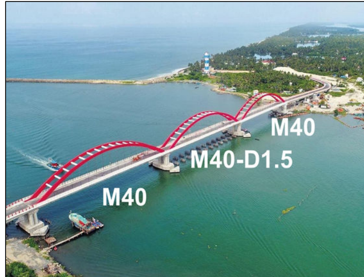
125 years service life Coastal Bridge, Kollam, Kerala
