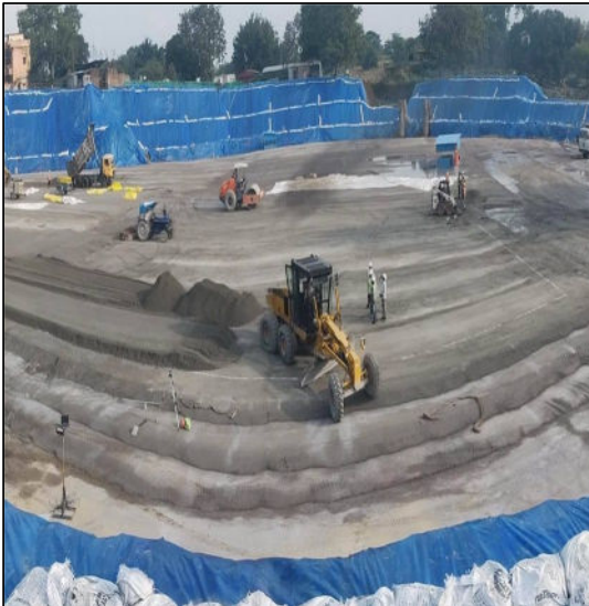
Concrete foundation (1000-year design life) Ayodhya
